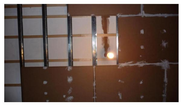
The PhoneStar boards are screwed to the resilient bars only using 25mm drywall screws. These screws must NOT penetrate into the ceiling. If possible fix the boards in a brickwork formation. Butt the boards tightly up to each other and to the perimeter walls. Ensure the PhoneStar board edges are sealed with PhoneStar Eco-tape after cutting to minimise sand spillage.
