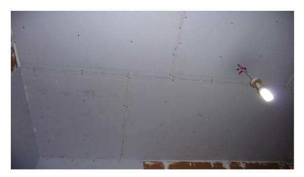
Acoustic plasterboard is then secured by screwing into the resilient bars only, using 38-42mm drywall screws. It is best to use a brickwork pattern. If you are only treating the ceiling and not the walls then leave a 5mm gap all around the perimeter edges and seal this gap with permanently flexible sealant. The joints and screw heads are then sealed as normal. In this case the ceilings and walls have both been upgraded to create an acoustic seal, so the plasterboard can go into the corners.
