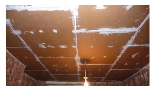
The PhoneStar boards can optionally be sealed with flexible sealant at the joints and perimeter, to ensure there are no gaps to allow sound to escape through. The screw heads are also sealed in this case.
