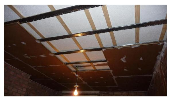
The existing plasterboard can be left in place. The ceiling is then battened to reduce the vibrations coming from the floor above. Flexible thermal insulation can optionally be placed between the battens. The resilient bars are then attached perpendicularly to the battens at 400mm centres. They must not quite touch the surrounding walls as this may cause flanking sound.
