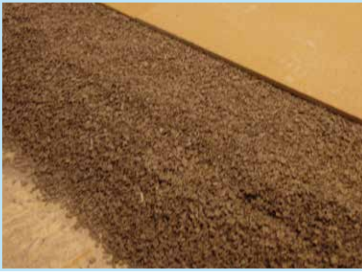
1. Cemwood levelling bed on OSB board - below wood fibre boards
