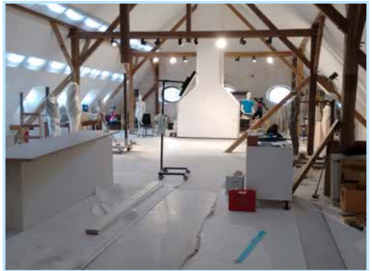
4. Studio with finished industrial type flooring
