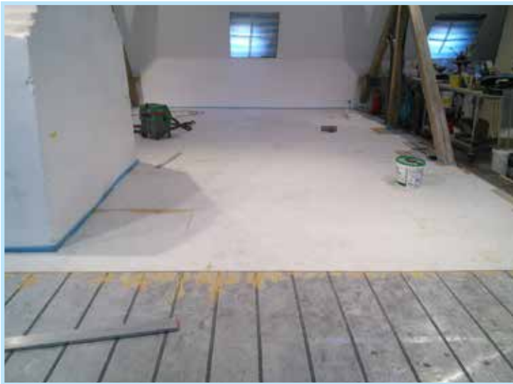
3. Decoupling plate bonded to PowerFloor Slimline UFH
